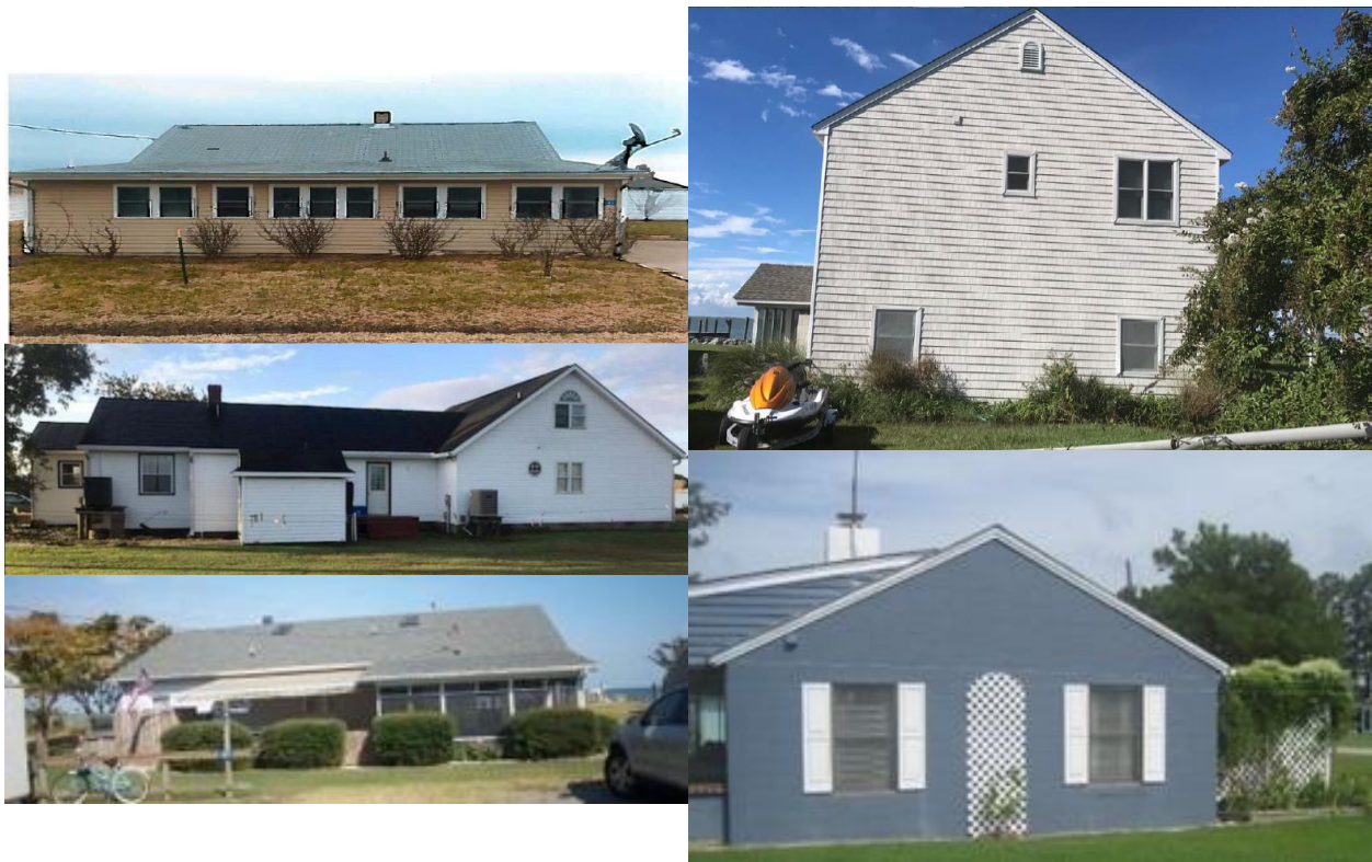
Figure 2: Mitigated properties pre-mitigation photos
