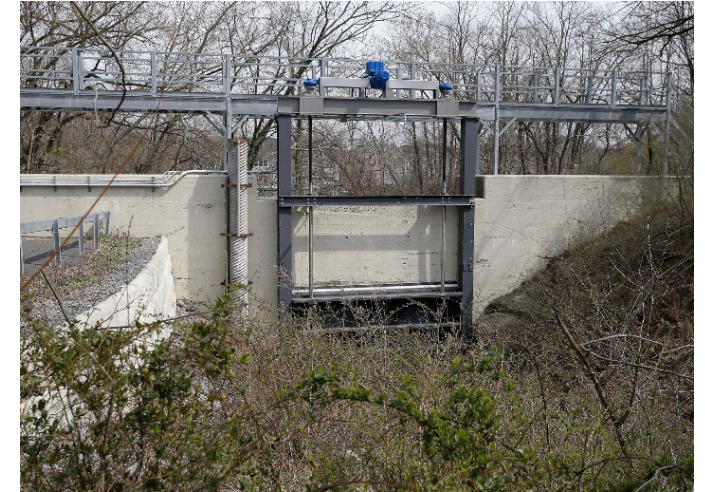
Bowman Dam sluice gate
